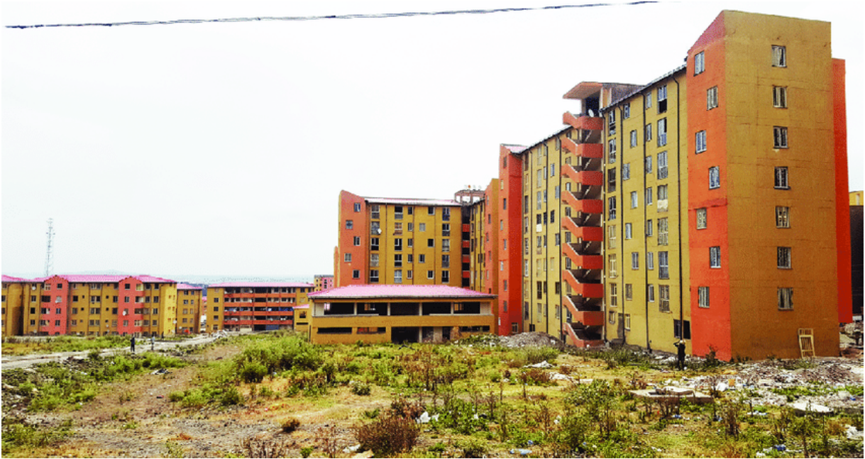
FIGURE 100 INCREMENTAL HOUSING IN ADDIS ABABA 86
