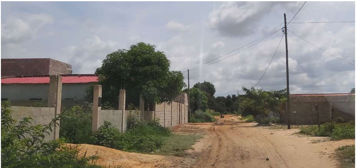
FIGURE 46 IMAGE OF A STREET IN VILA FLOR
