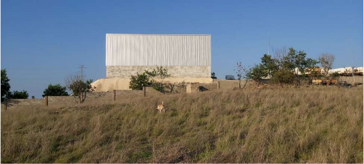
FIGURE 67 IMAGE OF THE DW SITE, LOOKING NORTH
