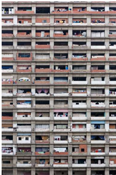
FIGURE 99 TORRE DAVID FAÇADE 85
