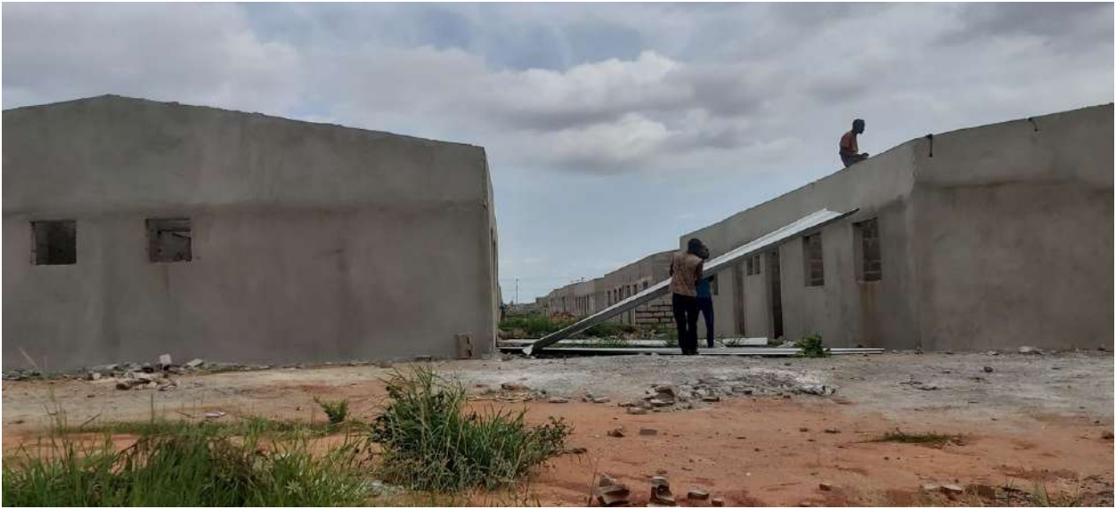
FIGURE 55 HOUSE BEING CONSTRUCTED IN THE ZANGO III NEIGHBORHOOD
