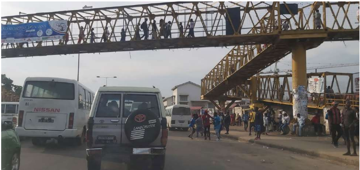
FIGURE 66 PEDESTRIAN BRIDGE ABOVE HIGHWAY
