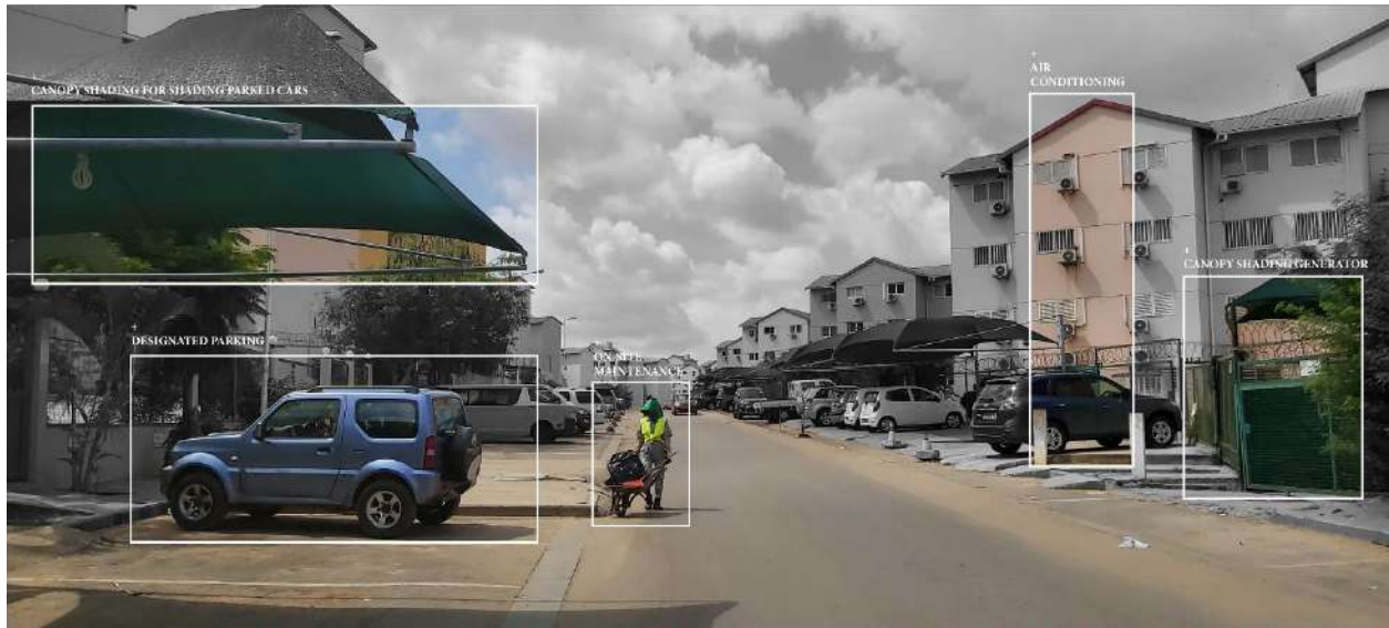
FIGURE 30 IMAGE ANALYSIS OF (PHASE 2) MULTI UNIT HOUSING IN NOVA VIDA SHOWING KEY ELEMENTS
