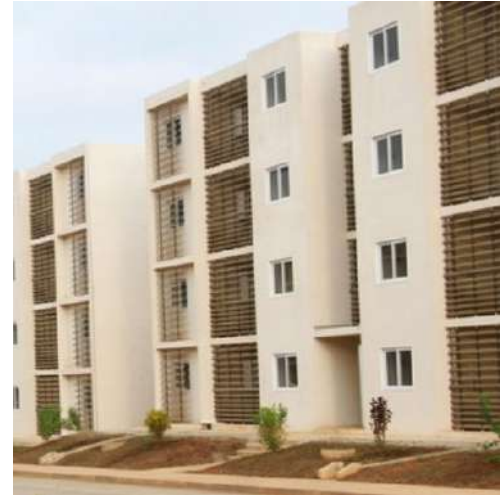
FIGURE 143 FLOOR-TO- CEILING BALCONY WITH LOUVRES IN THE KILUMOSO CENTRALITY IN UÍGE, ANGOLA
