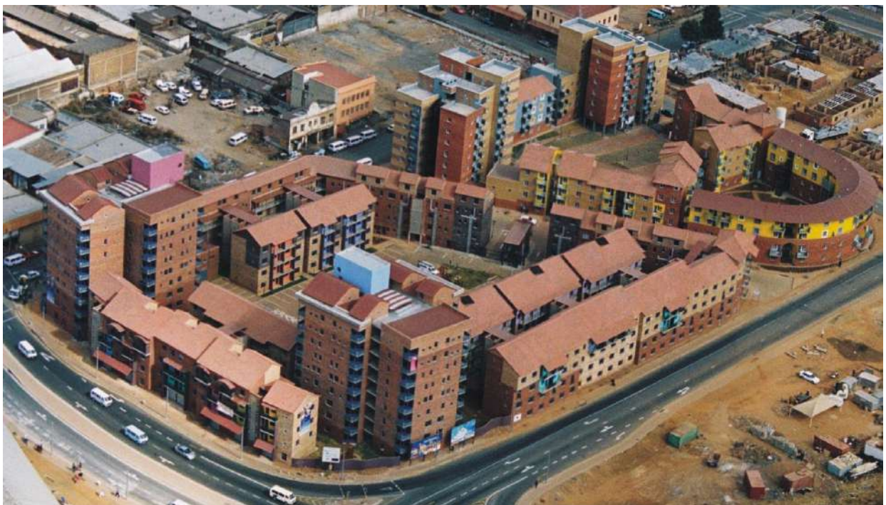
FIGURE 83 AERIAL VIEW OF BRICKFIELD 78
