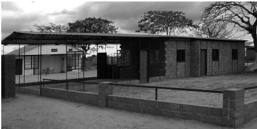
Figure 7.6 Incremental (Upgradeable) House in Zango
