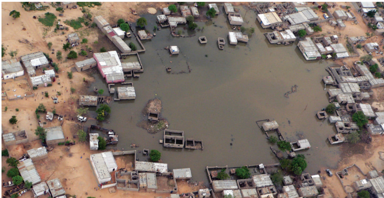
Permanently flooded basins due to poor drainage and impermeable soils © Development Workshop
