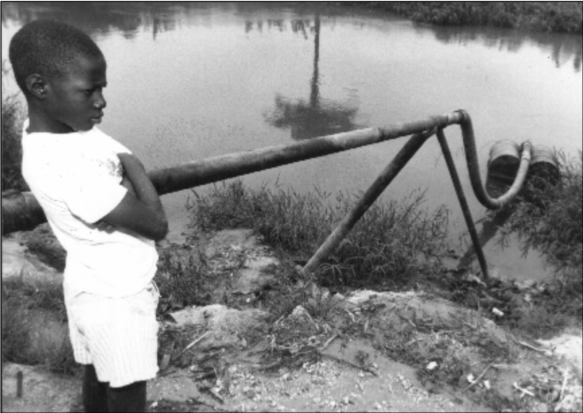
Water filling point at Kifangondo on the Bengo River.
