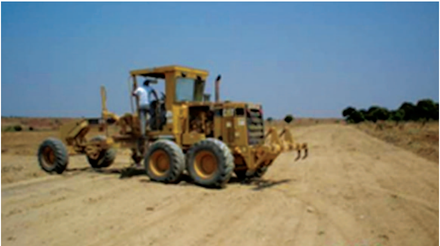
Preparing road clearances. © Development Workshop
